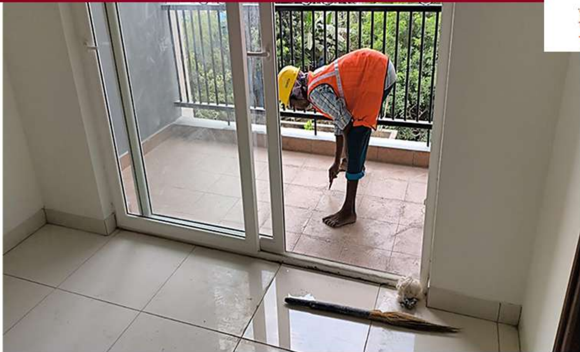
Block H Grouting Work in Progress
