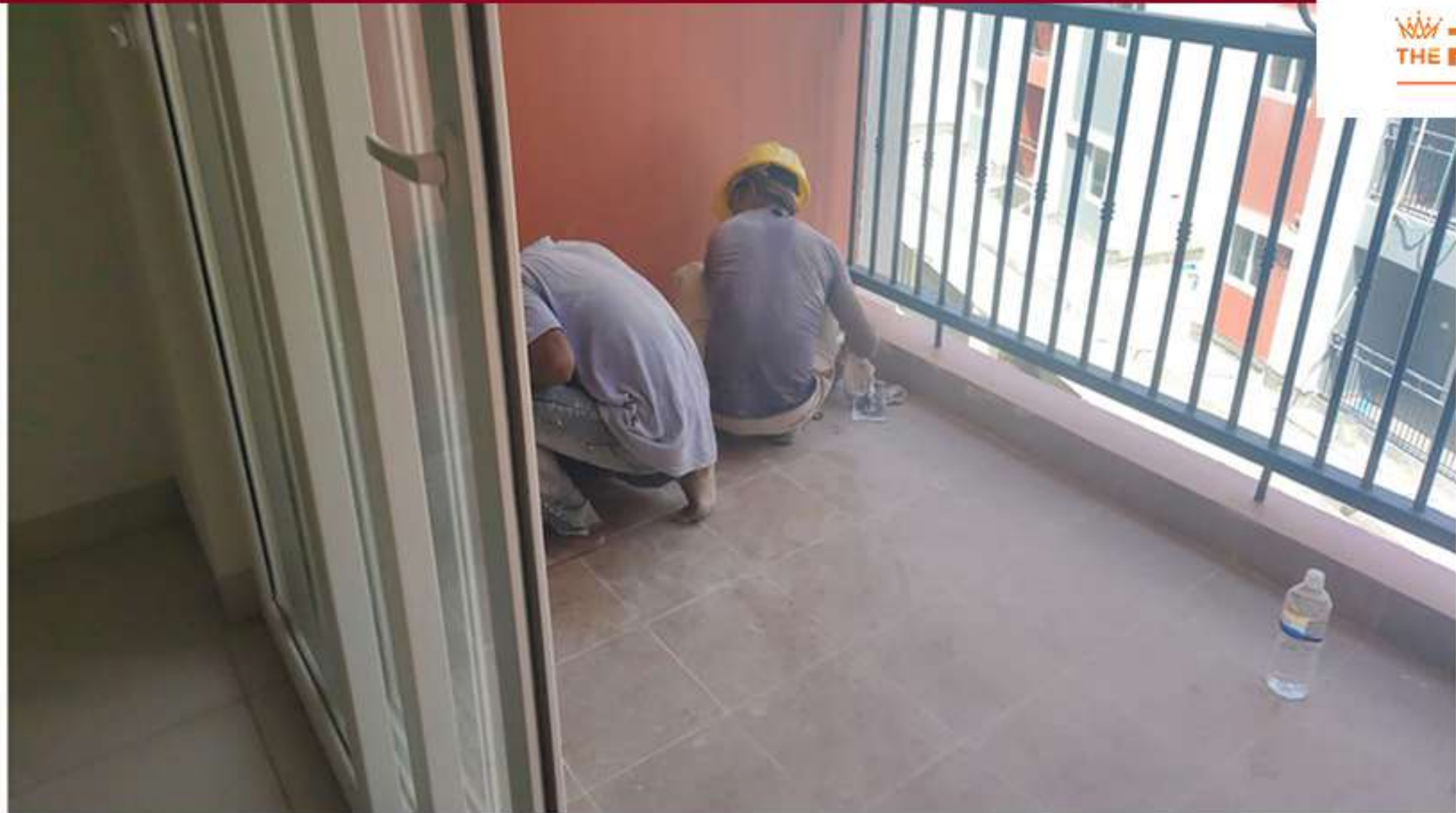
Cluster C Snag Work in Progress
