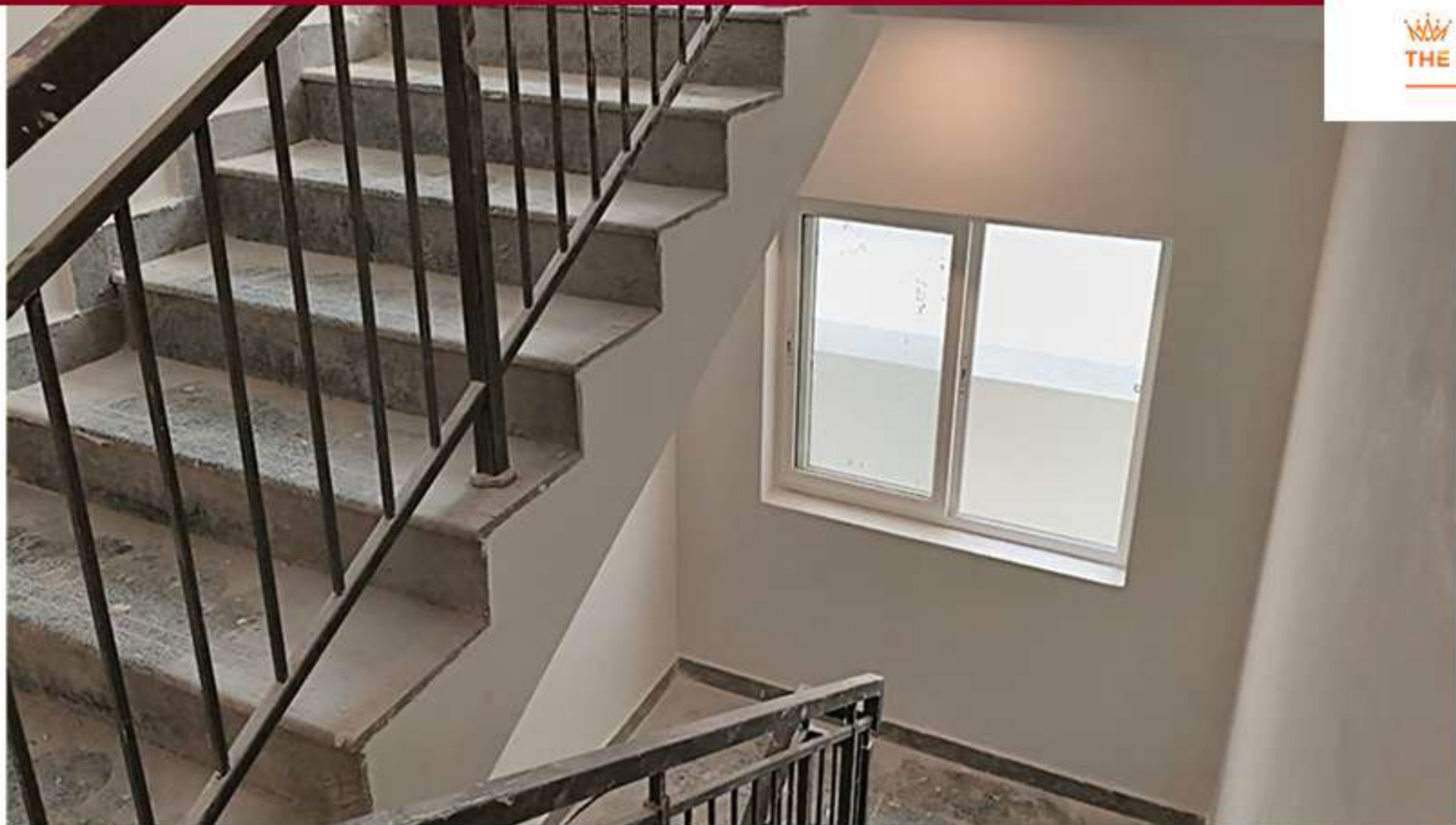
Cluster H & J Staircase Painting Work In Progress
