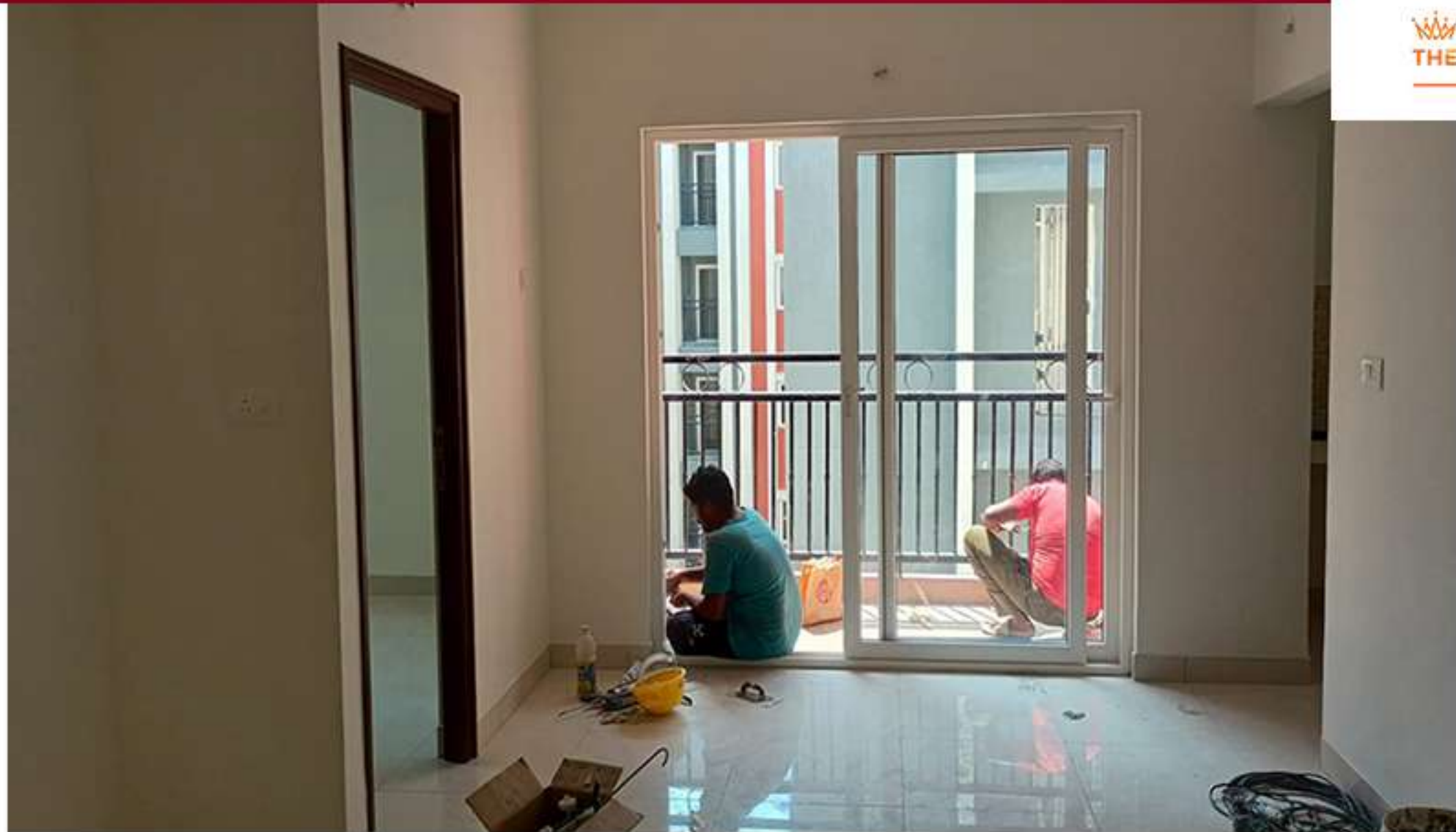
Cluster D Snag Work in Progress
