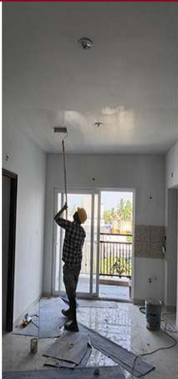
Cluster A Painting Work in Progress
