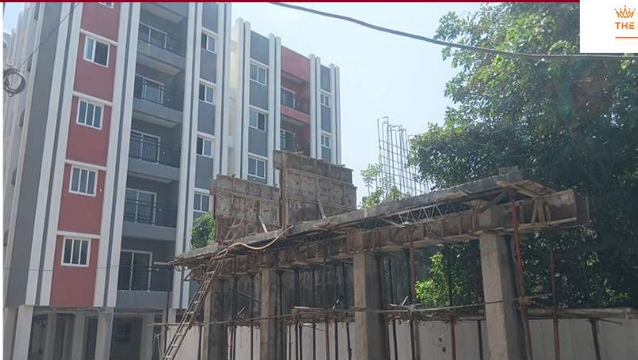
Transformer Yard Work in Progress
