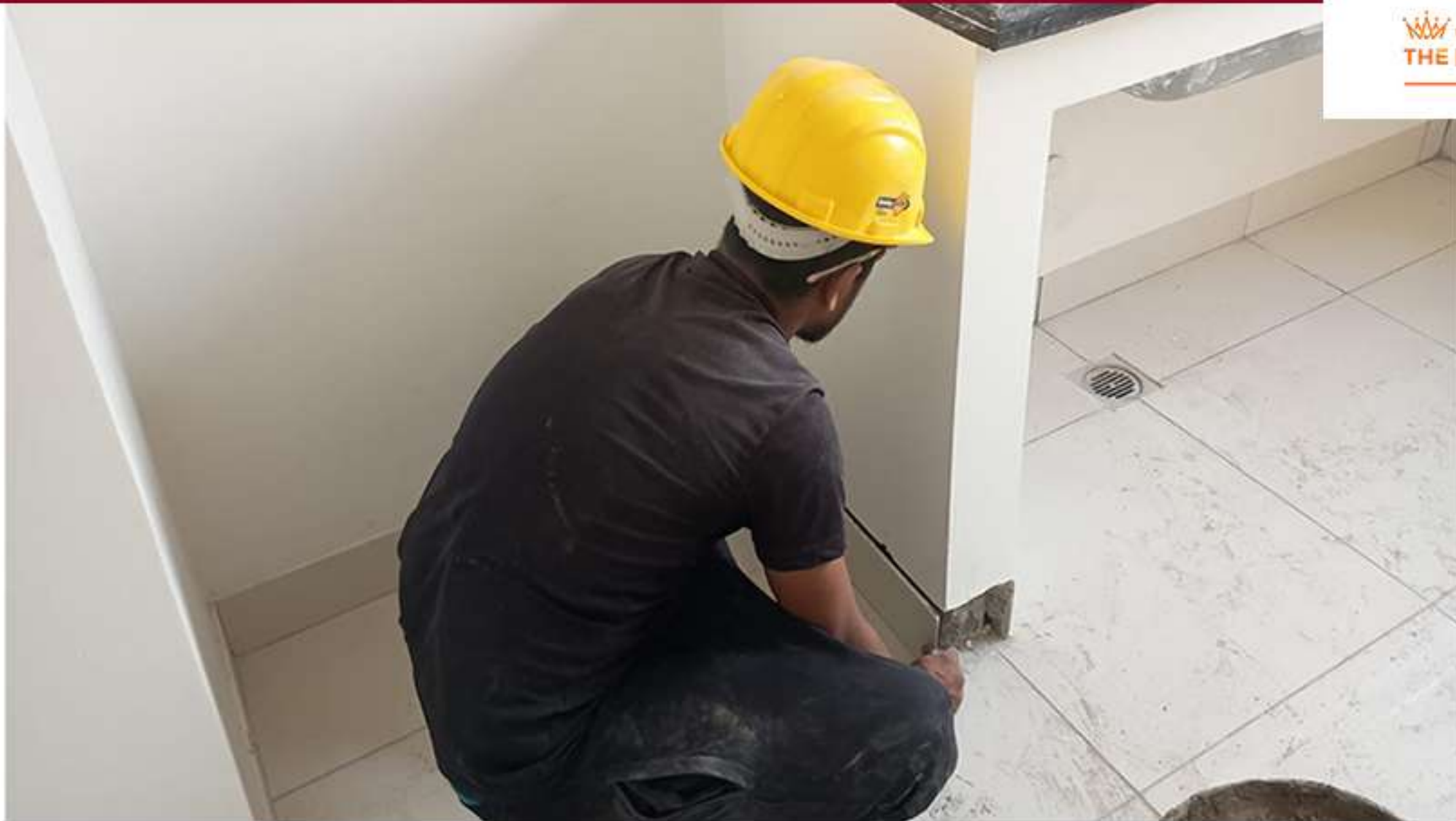
Cluster E Tile Snag Work In Progress
