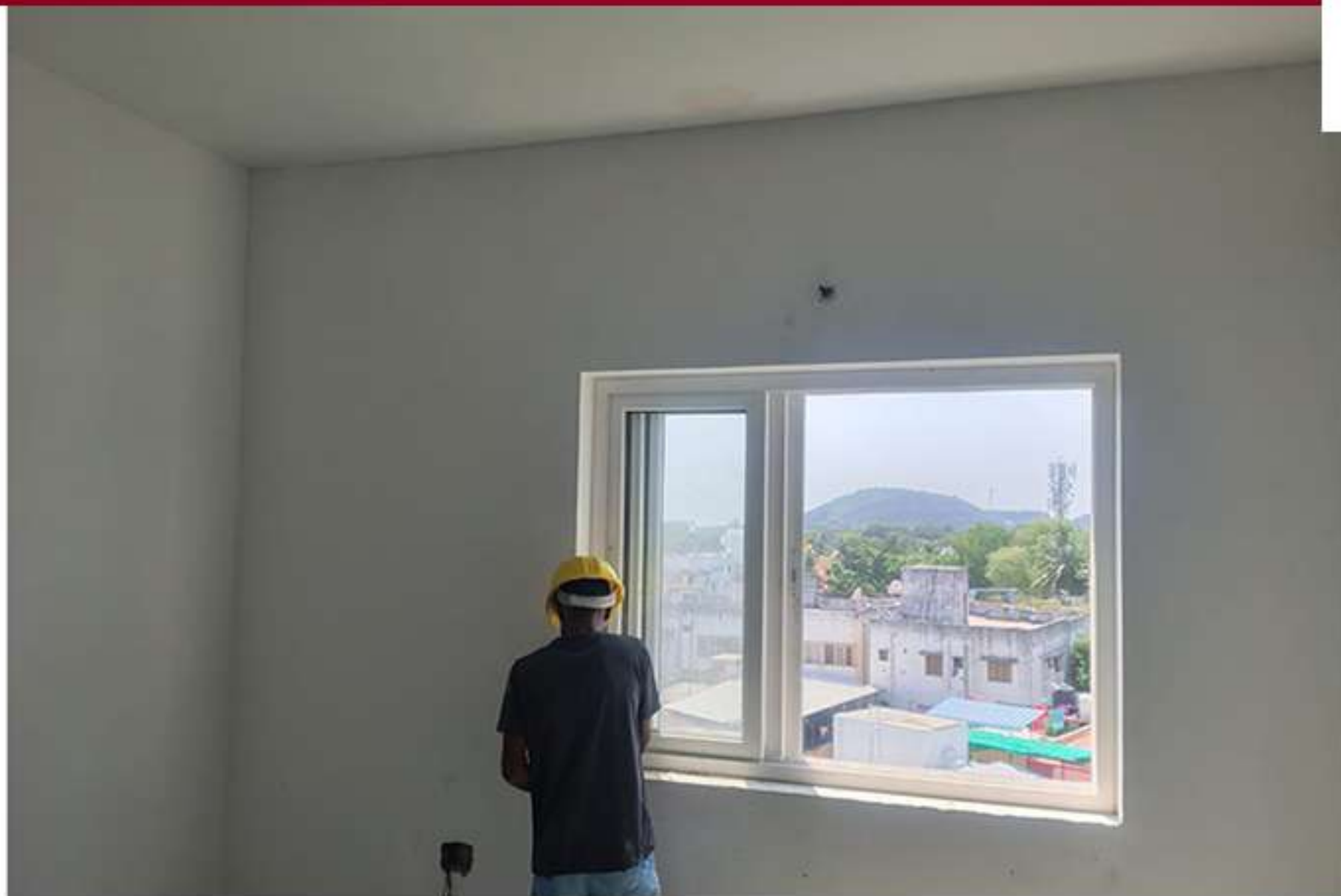
Cluster G Jams Correction Work in Progress
