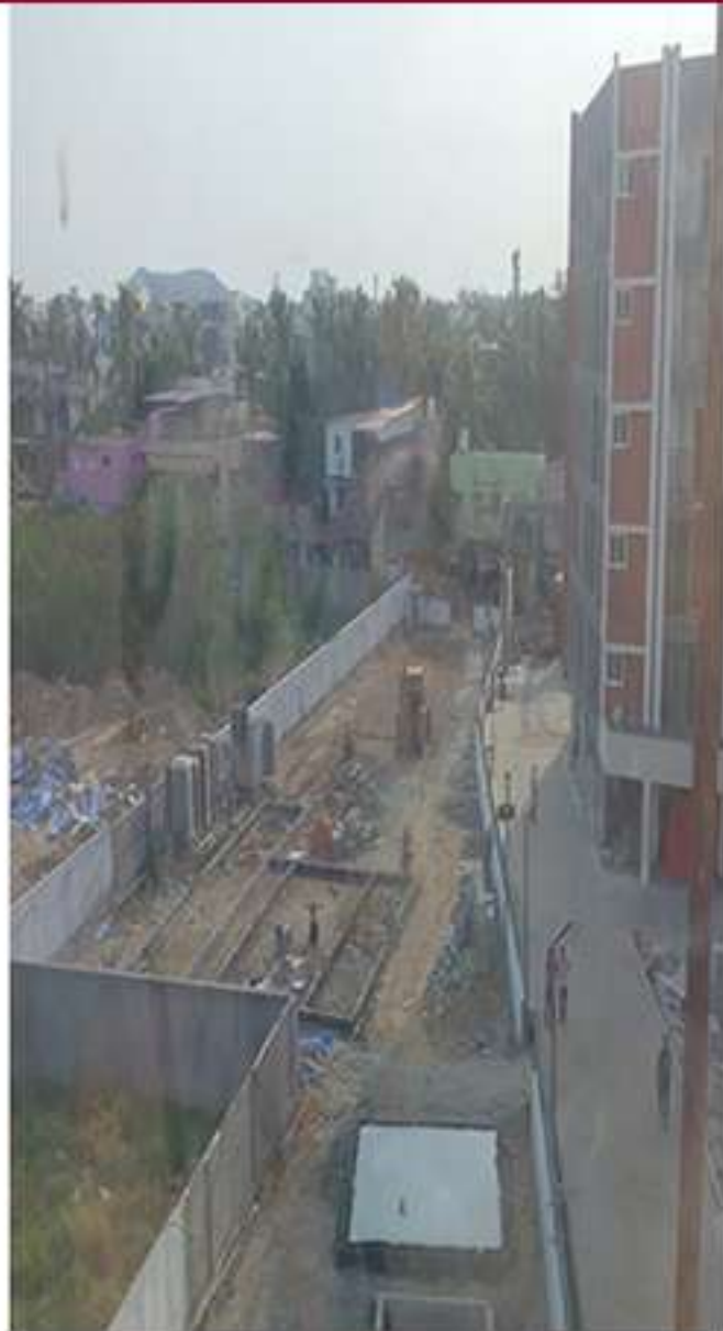
OSR Work In Progress
