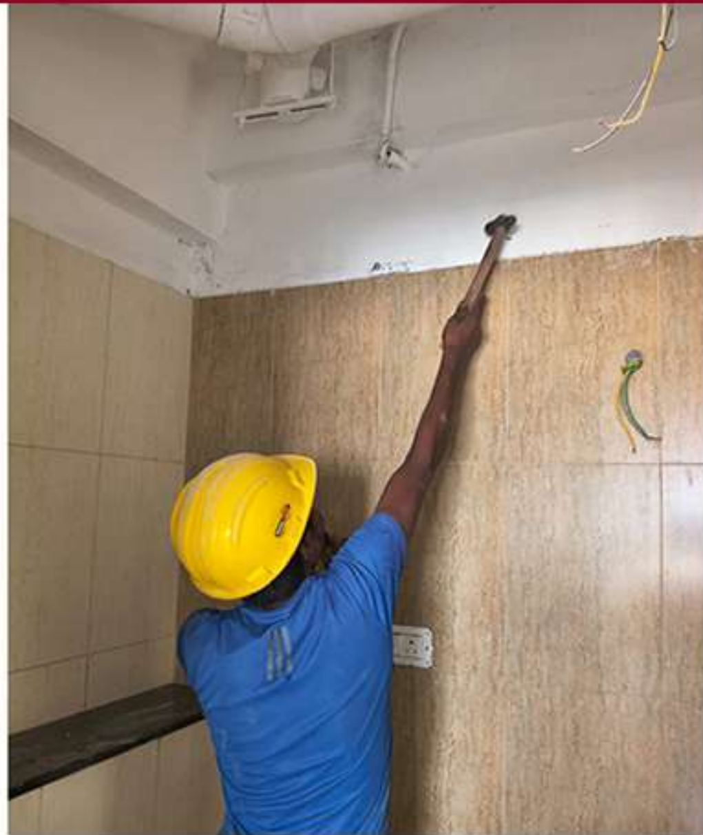
Cluster A False Ceiling Work in Progress
