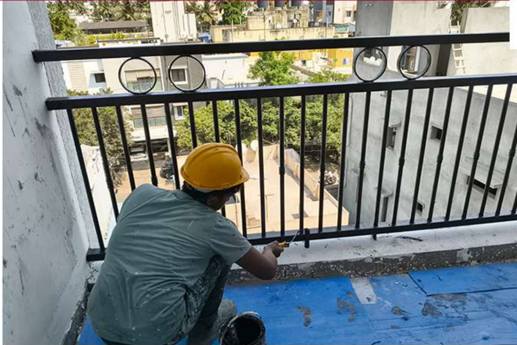
Cluster B Balcony Grill Painting Work in Progress
