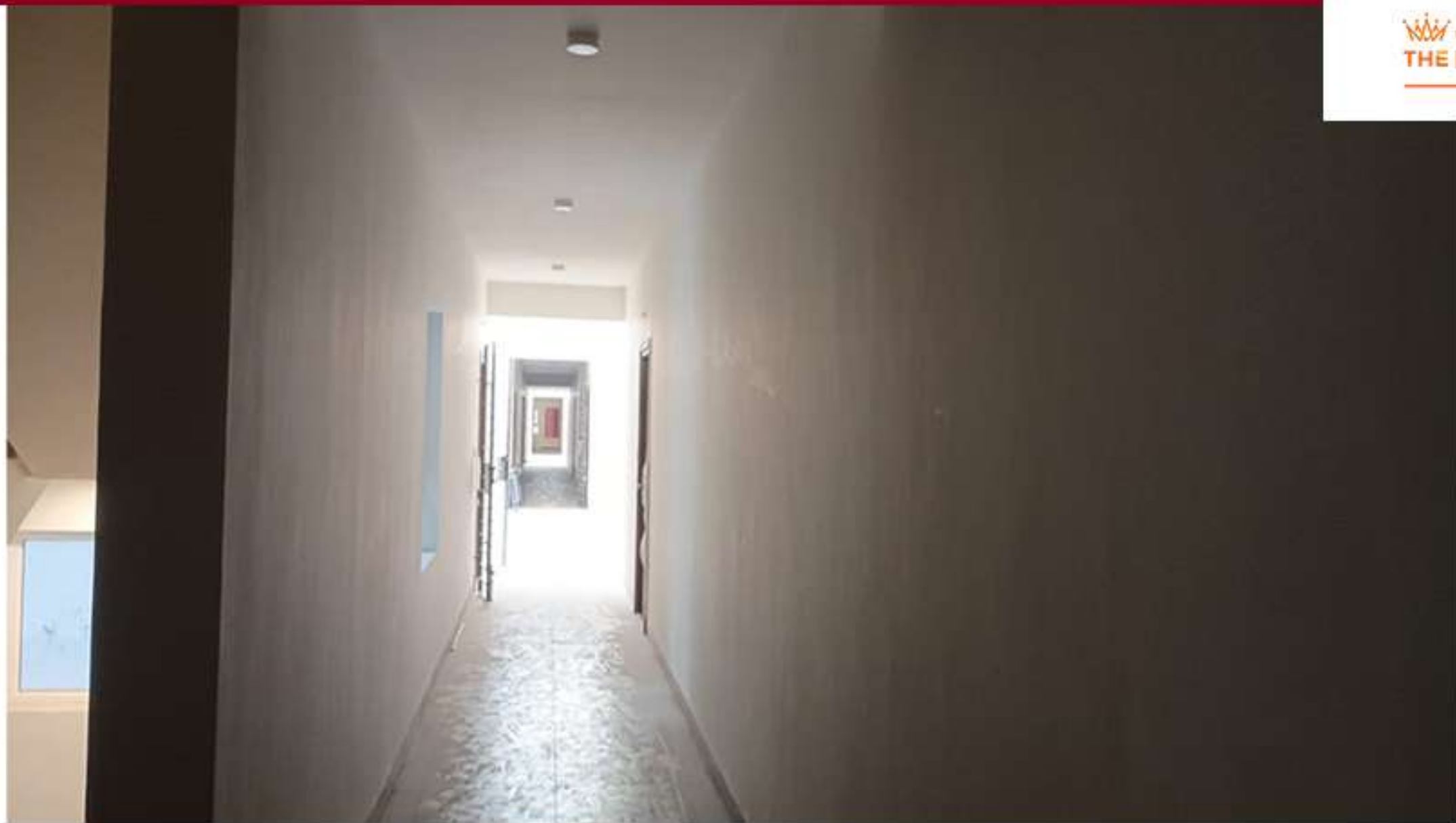
Cluster F Corridor Painting Work In Progress
