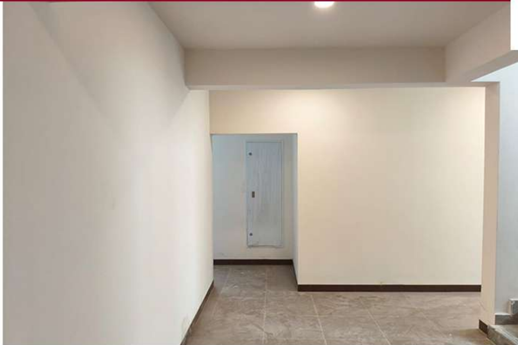
Cluster H & J Corridor Painting Work in Progress
