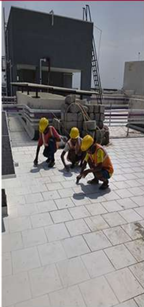
Cluster A Terrace Grouting Work in Progress
