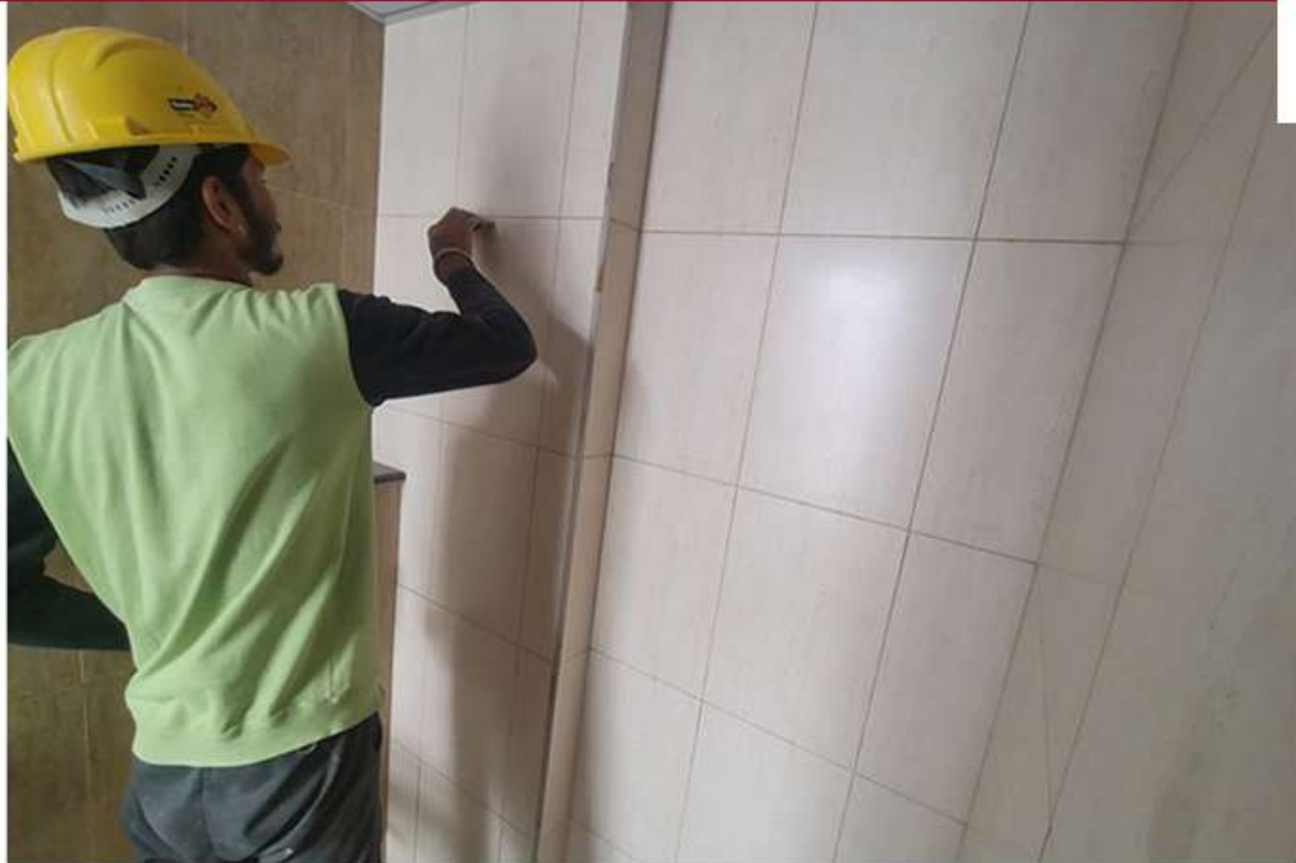
Cluster G Grouting Work in Progress
