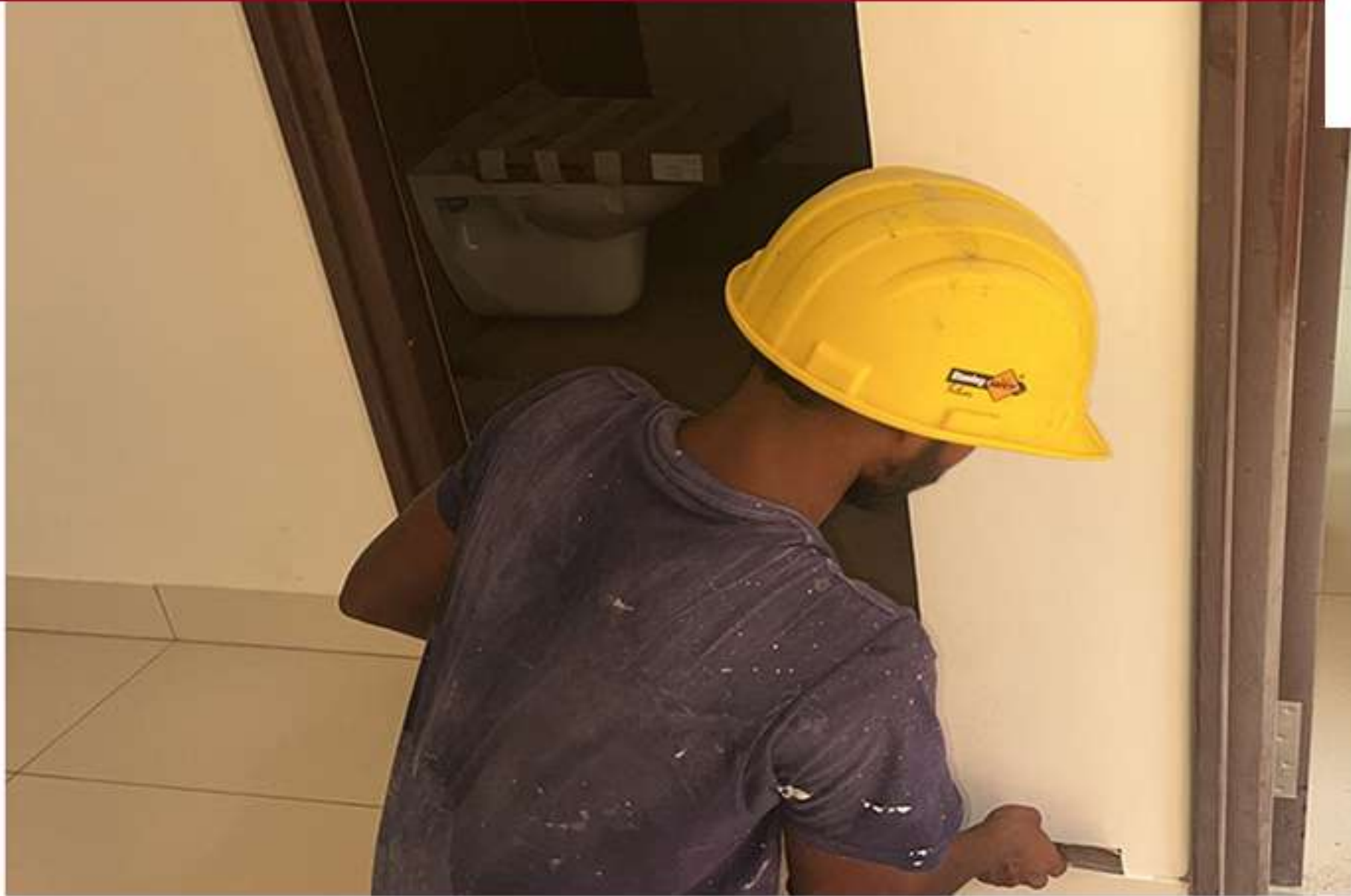
Cluster J Snag Work In Progress
