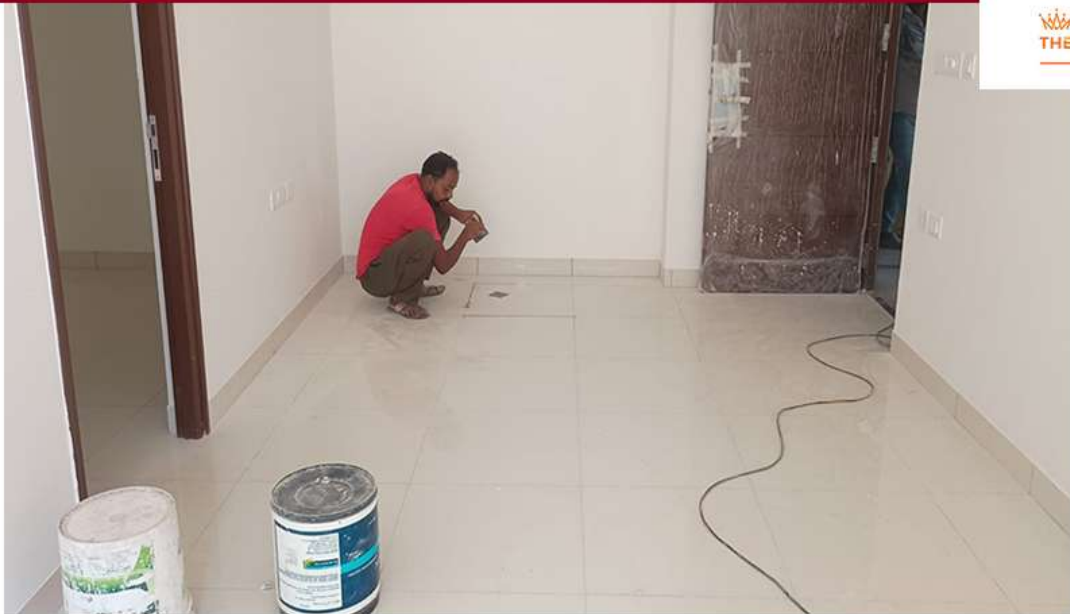
Cluster E Grouting Work in Progress
