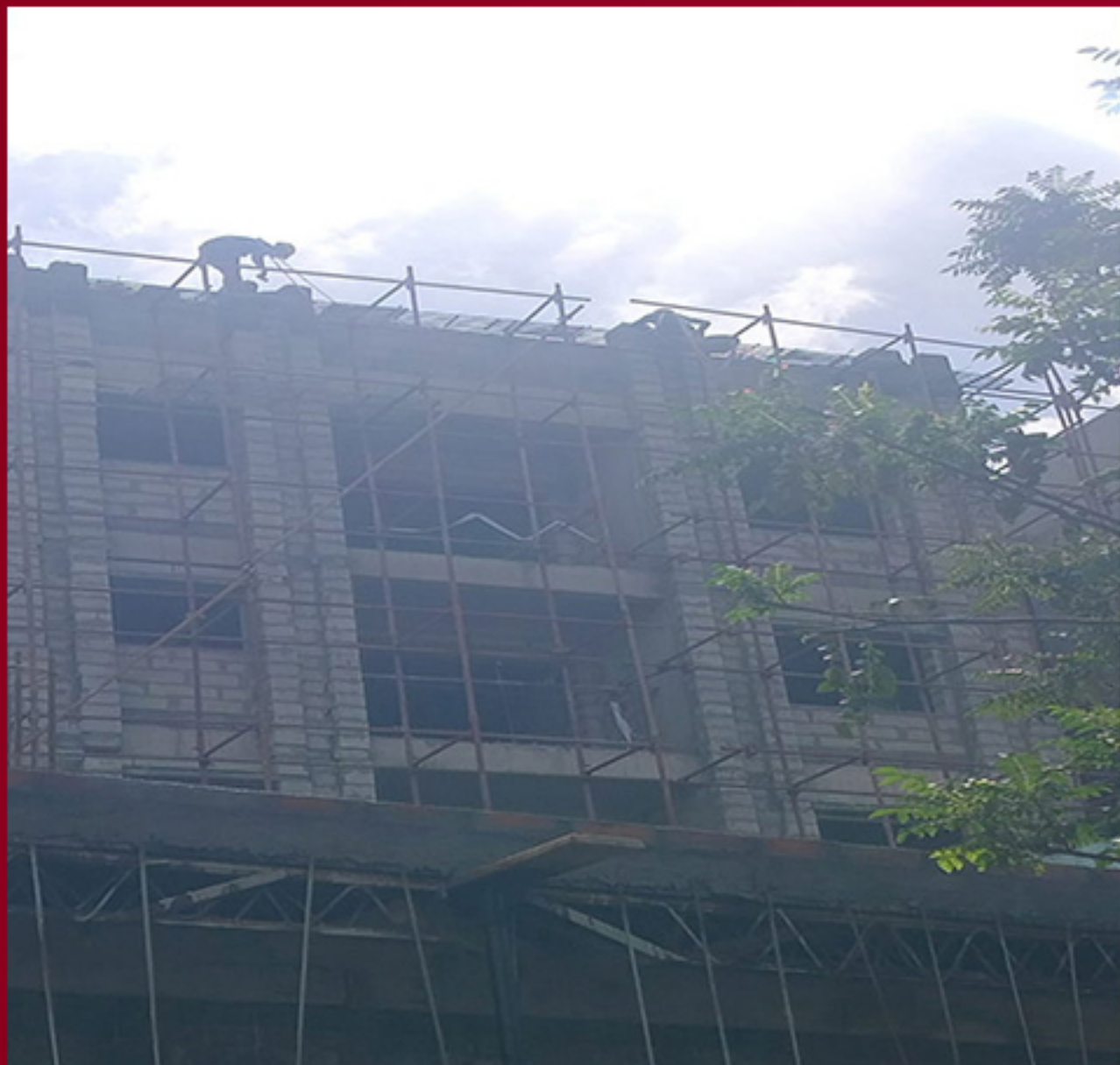
Block 1 – Cluster a west side external plastering work in progress
