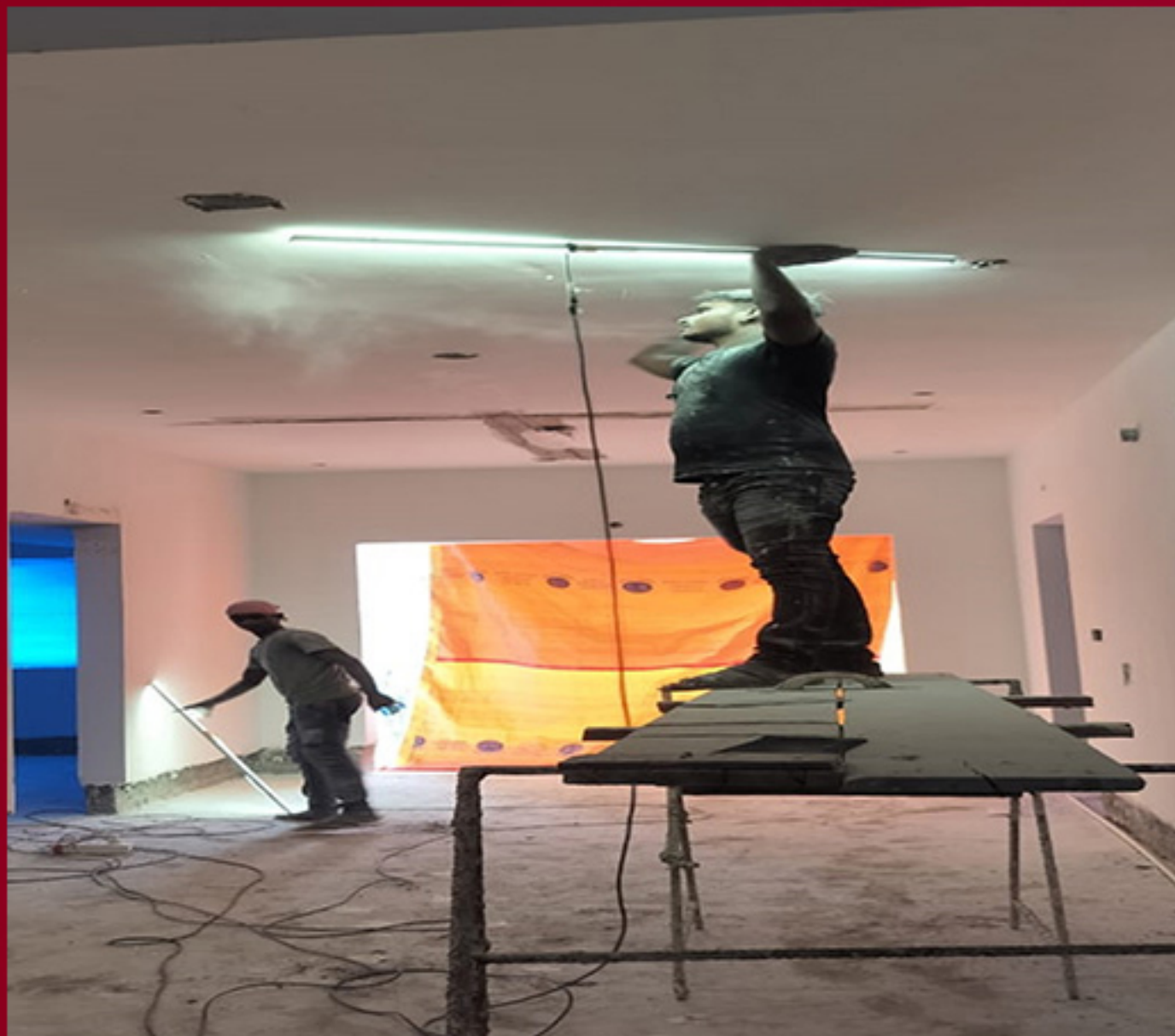
Block 1 – Cluster d ceiling & wall putty & primer work in progress
