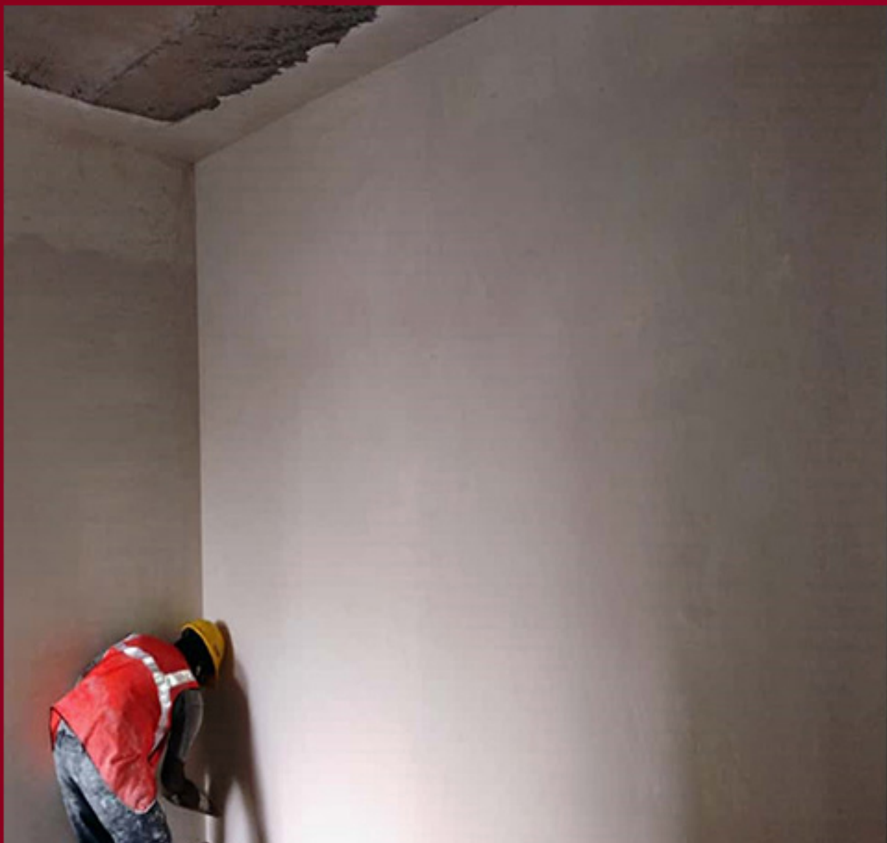
Block 1 – Cluster B 1 st floor gypsum work in progress
