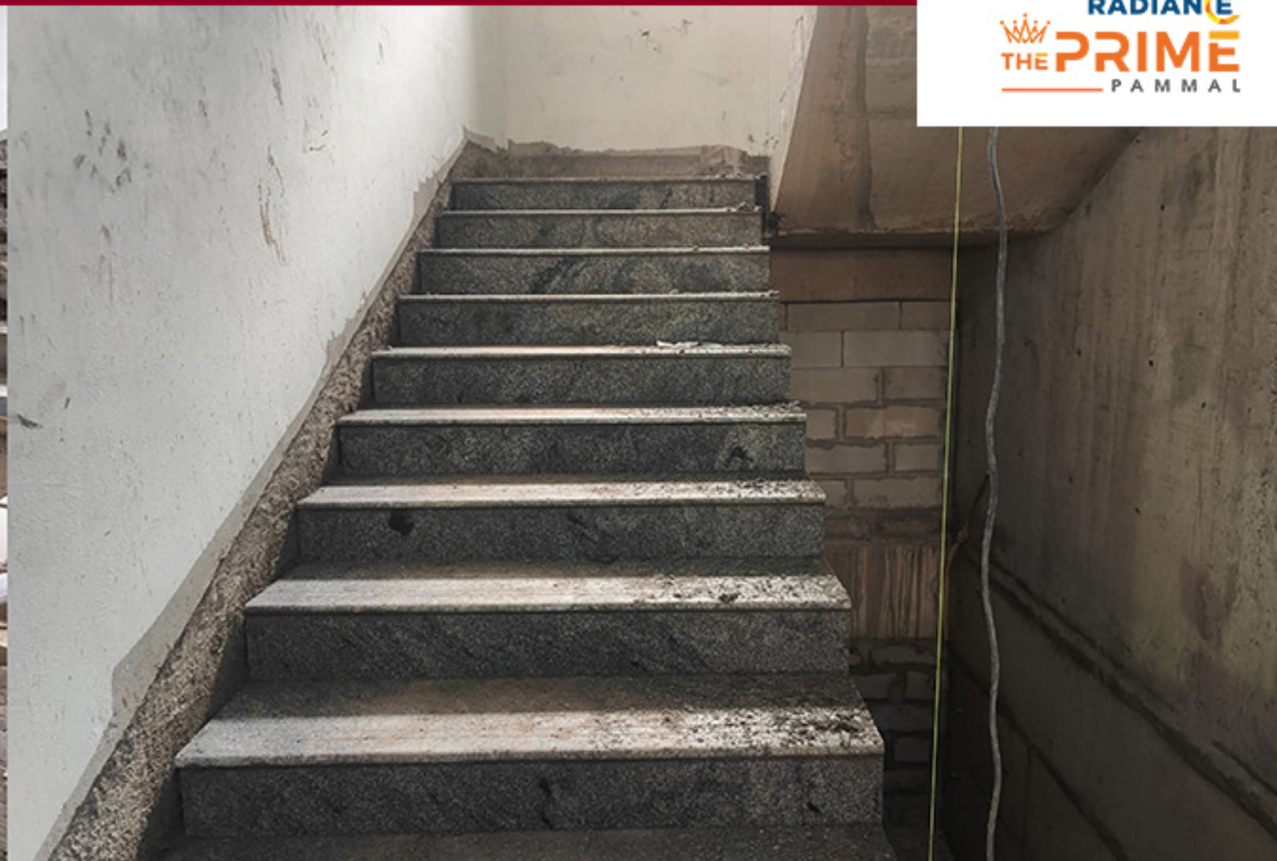
Block 1 – Cluster D tile laying work in progress
