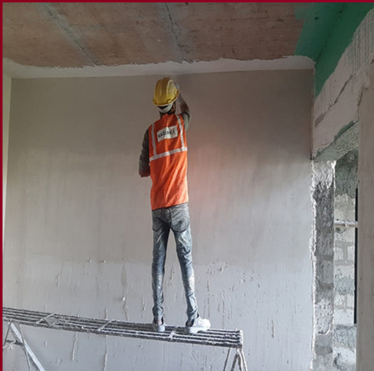
BLOCK 1 –CLUSTER C GYPSUM WORK IN PROGRESS
