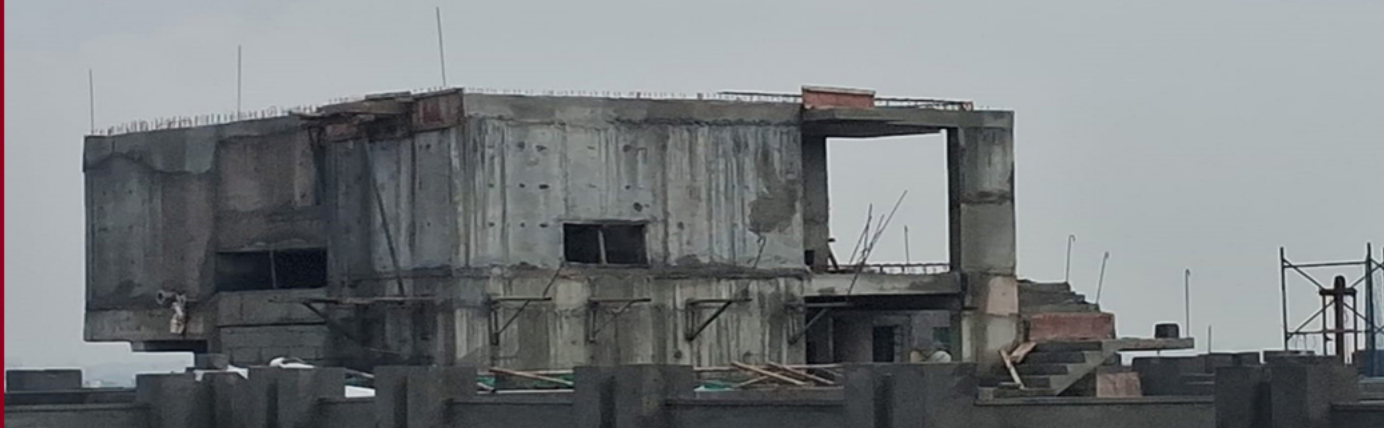
CLUSTER E OHT WALL CONCRETE COMPLETED
