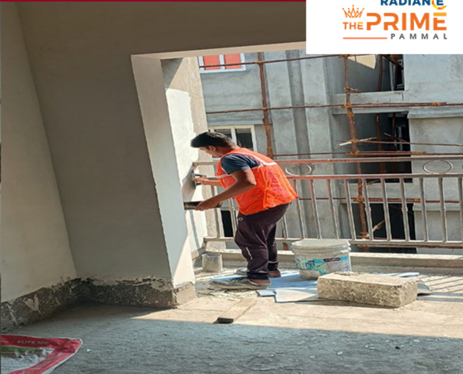
CLUSTER E CEILING & WALL PUTTY WORK IN PROGRESS
