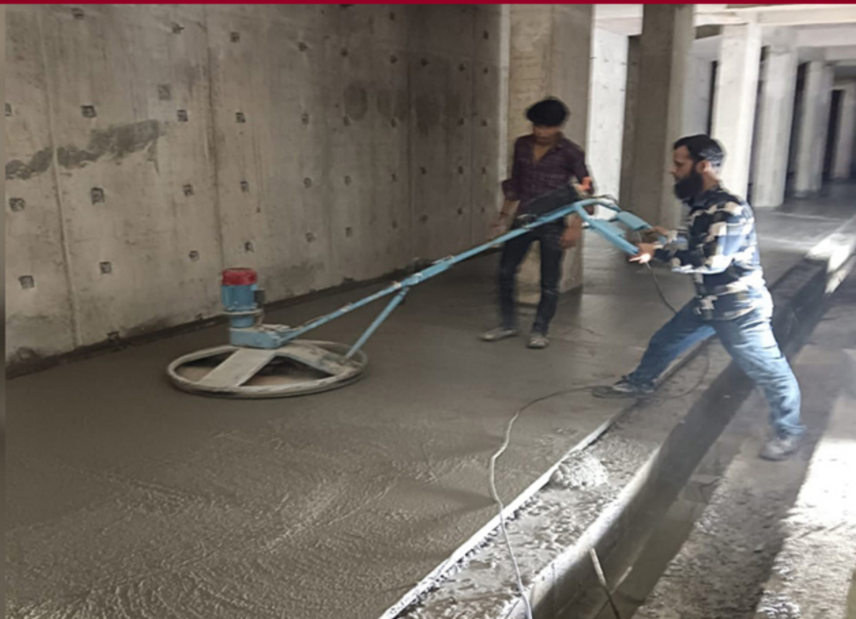
BASEMENT SCREED CONCRETE WORK IN PROGRESS
