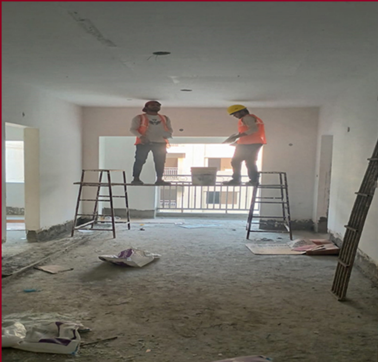
CLUSTER E CEILING & WALL PUTTY WORK IN PROGRESS
