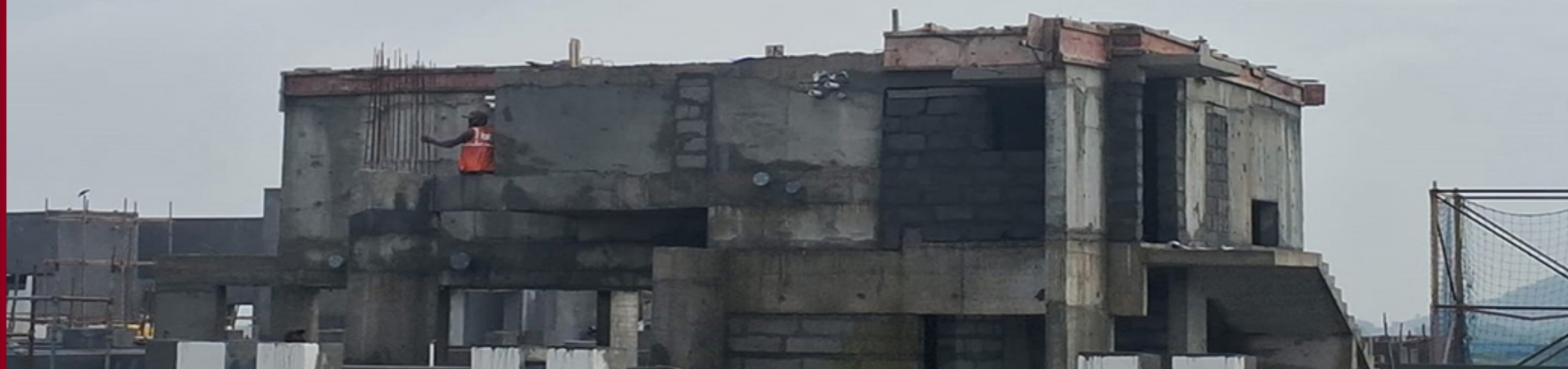
BLOCK 1 -CLUSTER F OHT WALL COMPLETED
