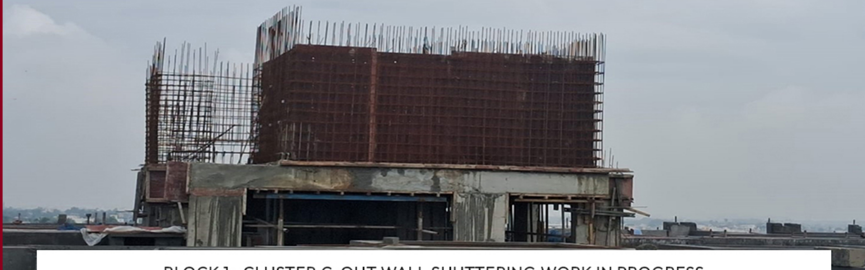
BLOCK 1 -CLUSTER C OHT WALL SHUTTERING WORK IN PROGRESS
