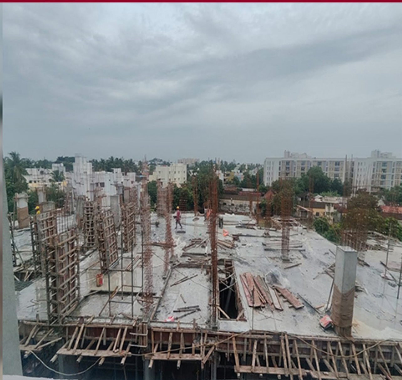
BLOCK 2 -CLUSTER G 4TH FLOOR COLUMN CONCRETE WORK IN PROGRESS
