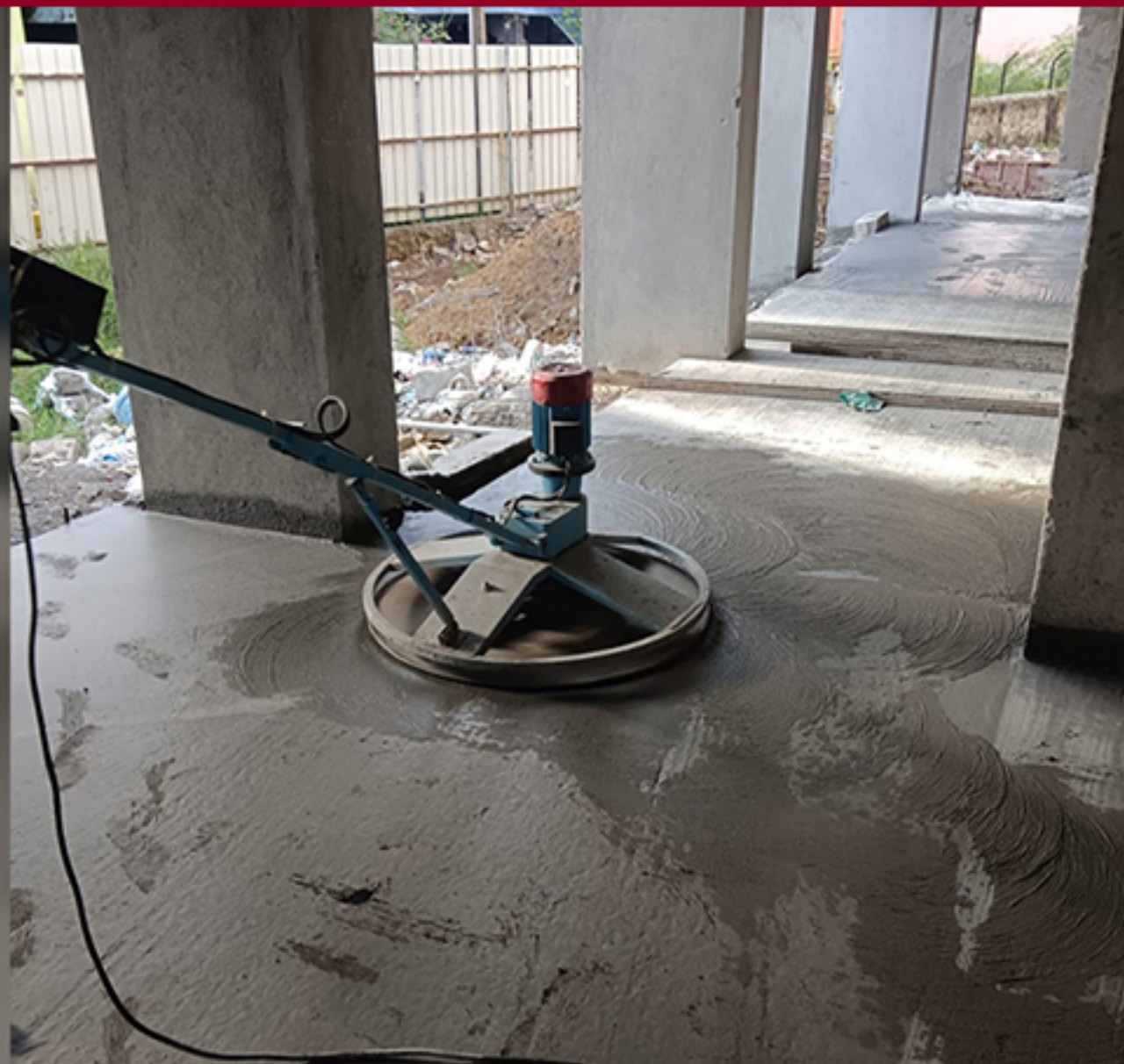
BLOCK 3 –CLUSTER H & J GRANO FLOORING WORK IN PROGRESS
