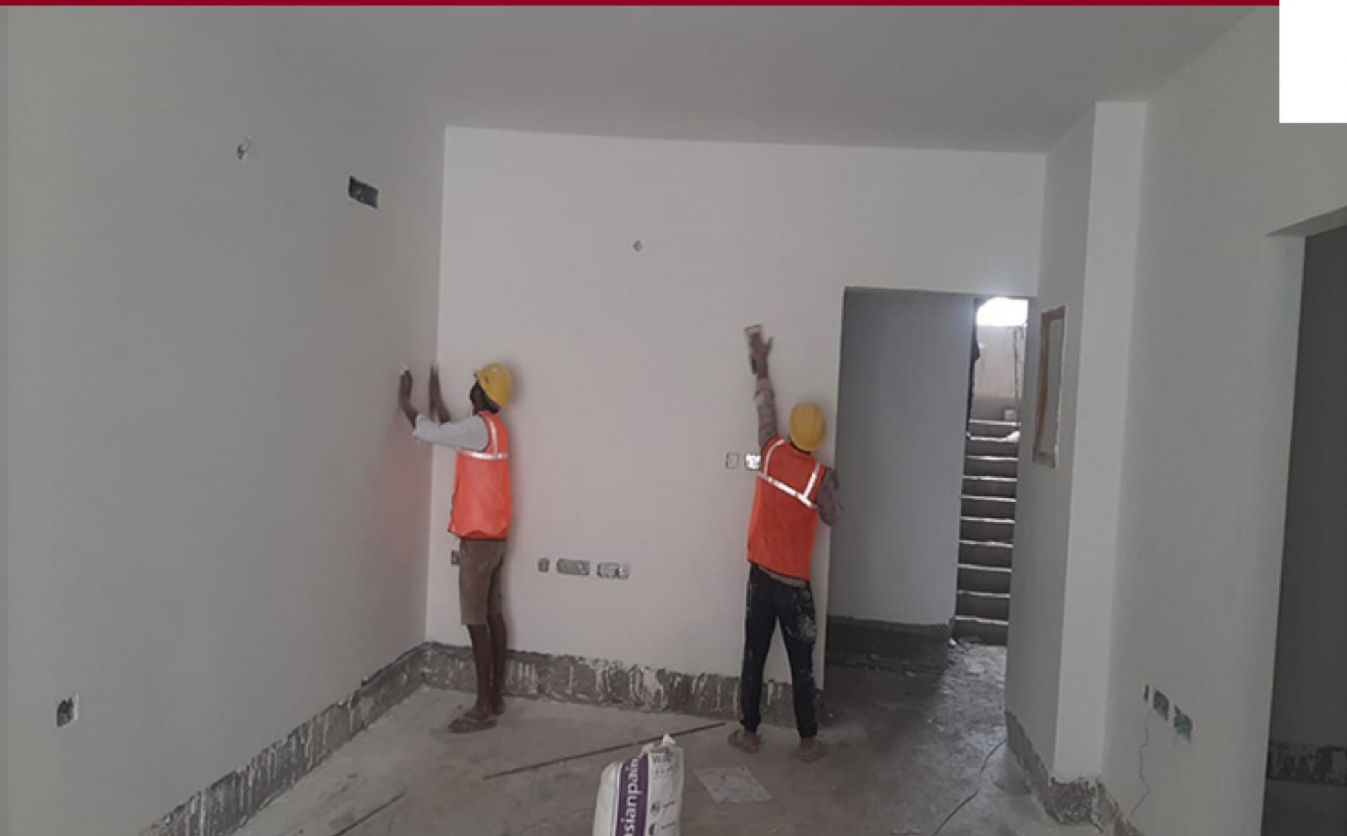
BLOCK 1 -CLUSTER D CEILING & WALL PUTTY WORK IN PROGRESS
