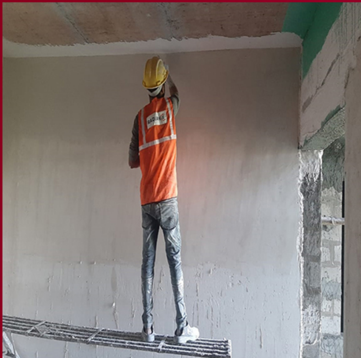
BLOCK 1 –CLUSTER C GYPSUM WORK IN PROGRESS
