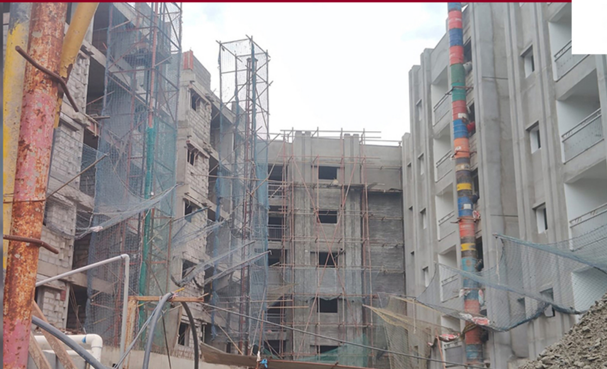
BLOCK 1 -CLUSTER C SOUTH SIDE EXTERNAL PLASTERING WORK IN PROGRESS
