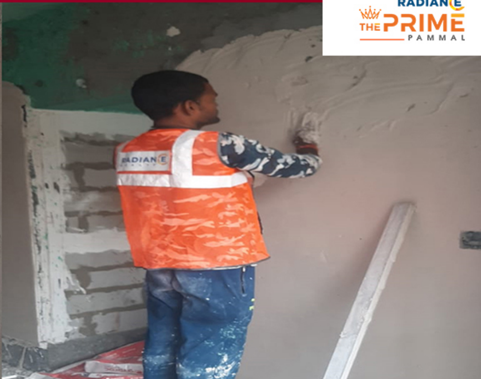
BLOCK 1 –CLUSTER C GYPSUM WORK IN PROGRESS
