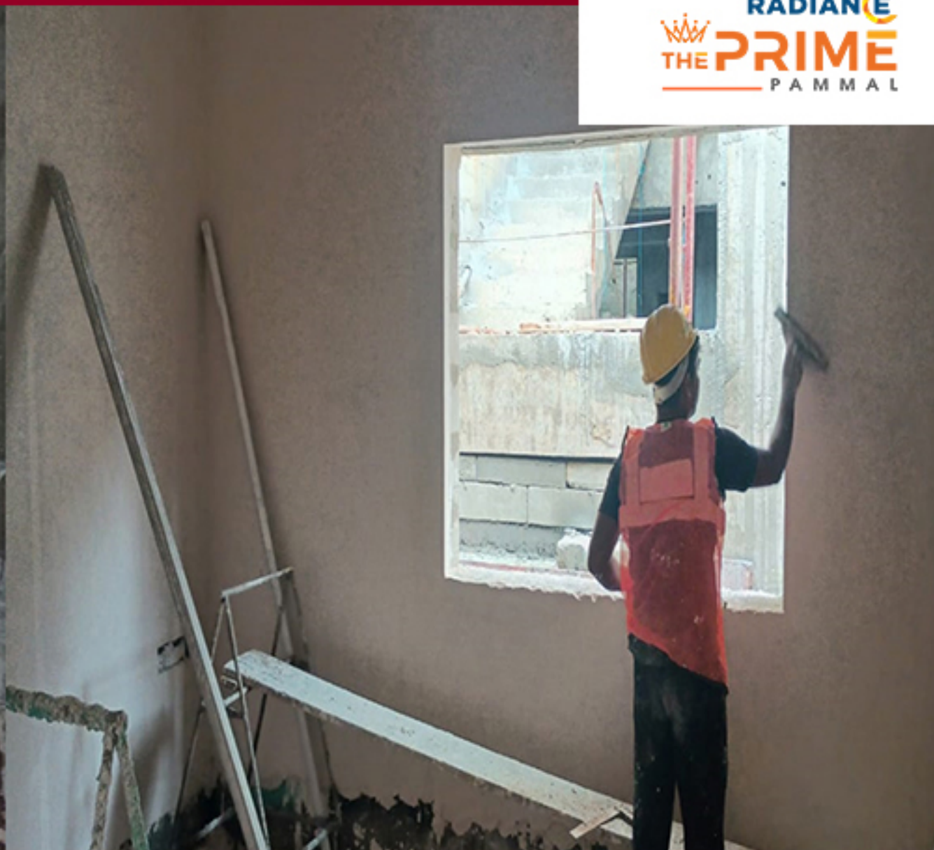
CLUSTER E PUTTY & GYPSUM WORK IN PROGRESS
