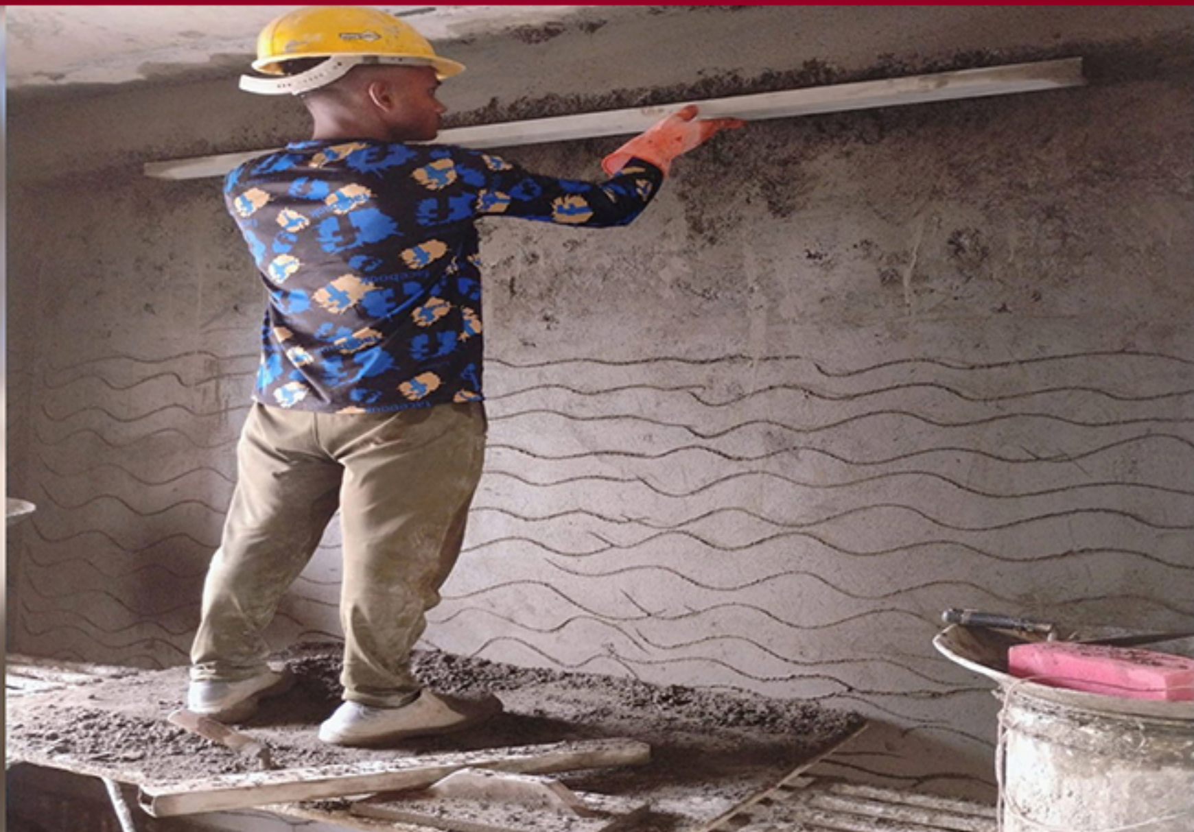
BLOCK 1 –CLUSTER A 1ST FLOOR TOILET WALL PLASTERING WORK IN PROGRESS
