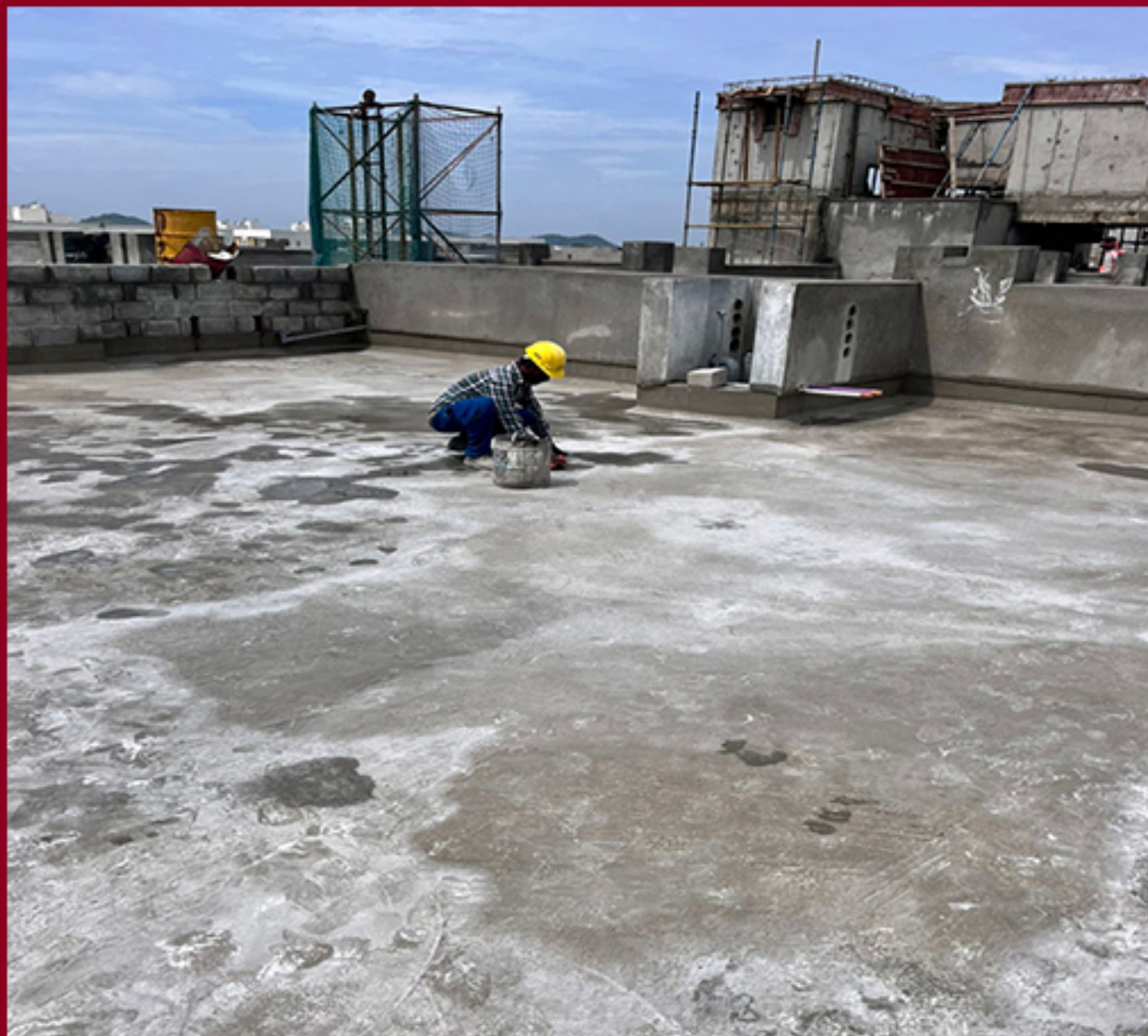
BLOCK 3 –CLUSTER H & J TERRACE CLEANING & WATERPROOFING WORK IN PROGRESS
