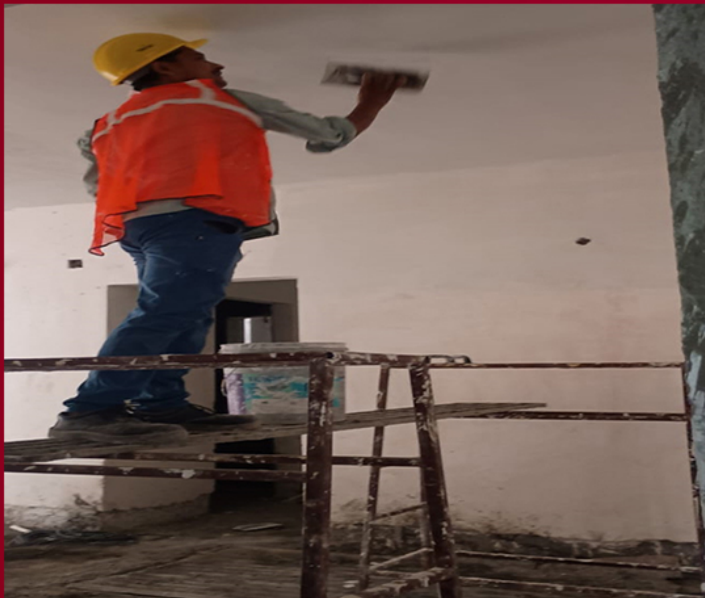
CLUSTER E PUTTY & GYPSUM WORK IN PROGRESS
